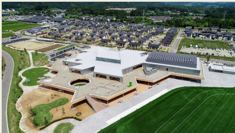
Figure 3.4. Exterior of the Manabiya Yumenomori School
